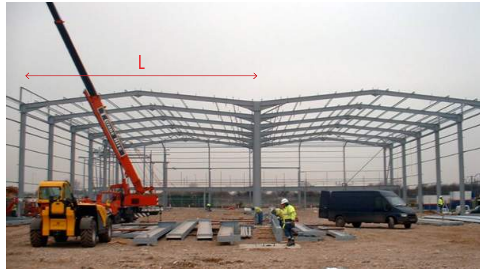
Example steel frame for an industrial building.
