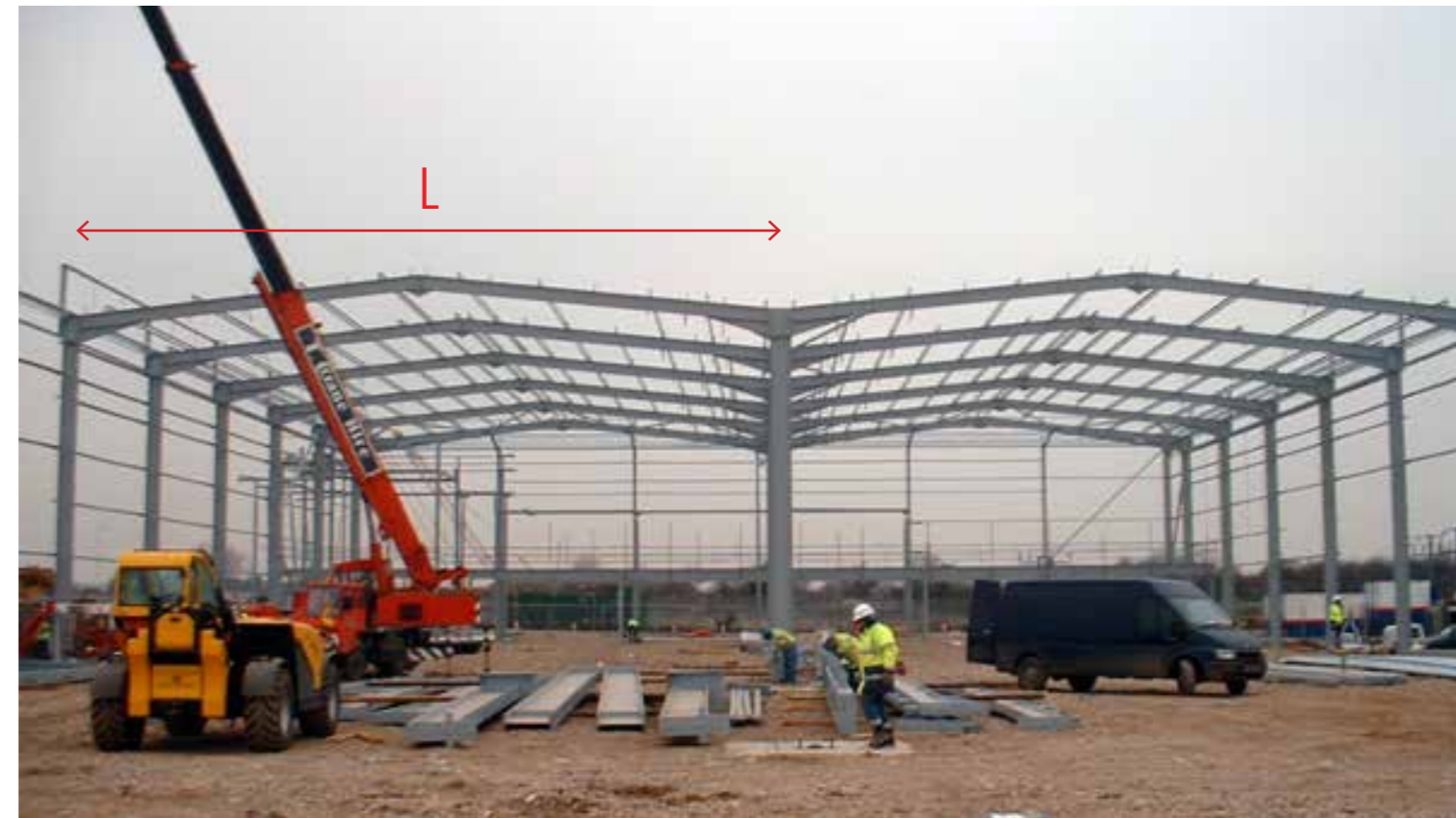
Example steel frame for an industrial building.
