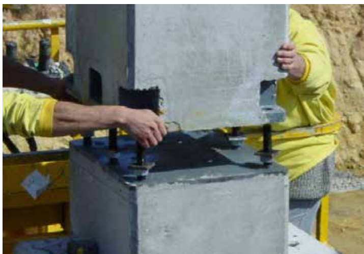
Peikko website image: concrete bolted connection during erection.
