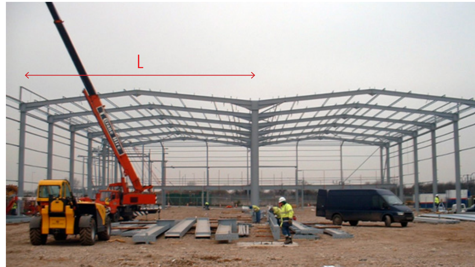
Example steel frame for an industrial building.
