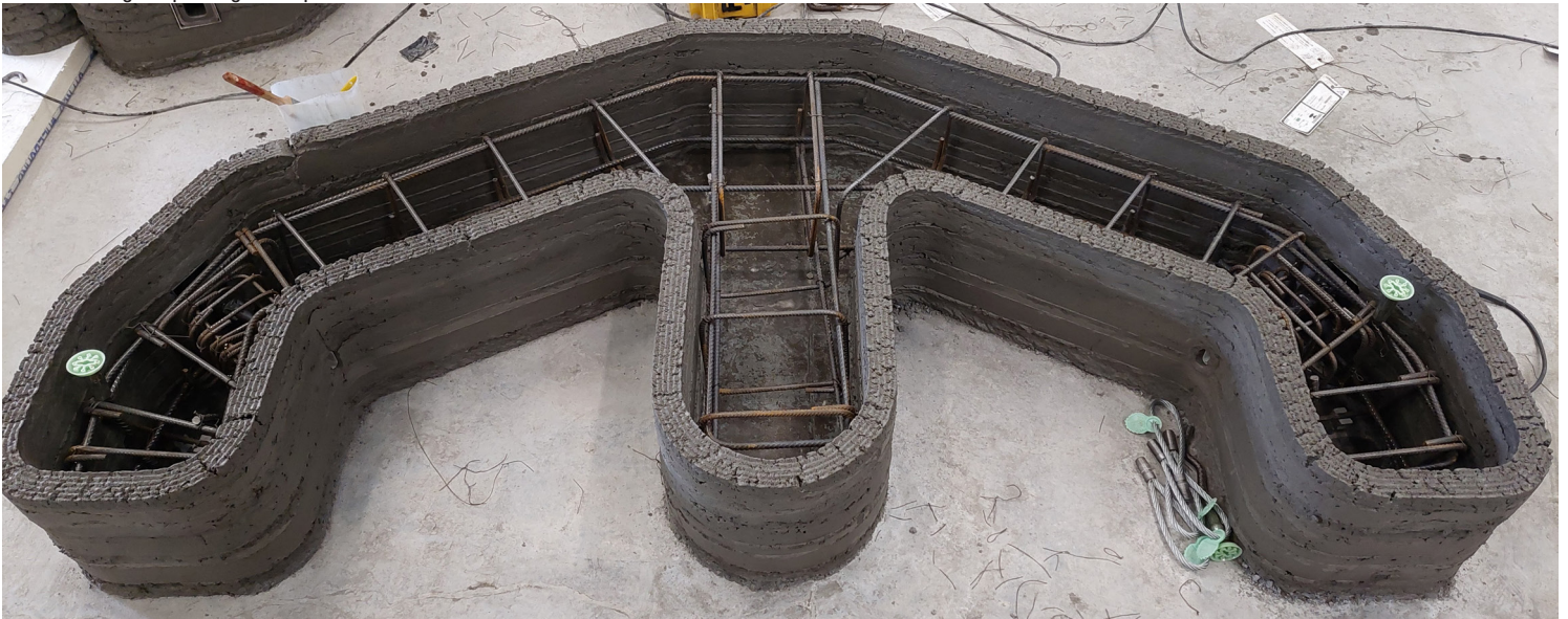
reinforcement within the printed perimeter
