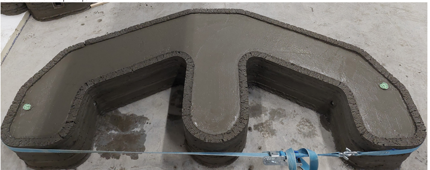
conventional concrete poured within the permanent formwork
